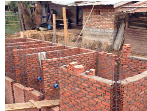
Construction of Anaerobic Baffled Reactor
