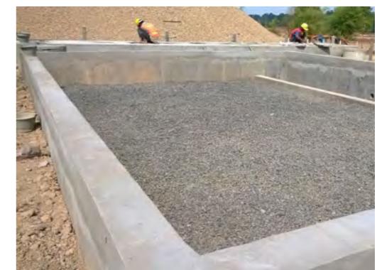
Construction of the Planted Gravel Filter
